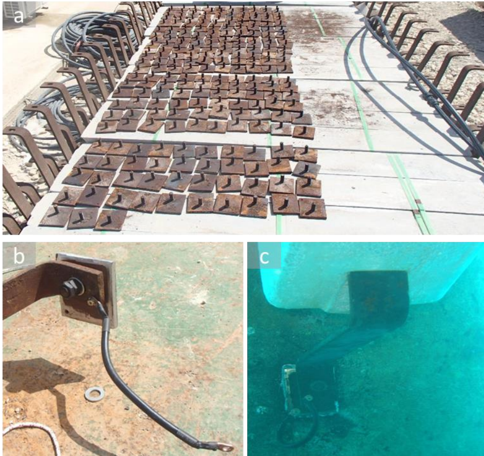
Figure 3. (a) The anodes and the metal plates, (b) the copper wire, and (c) as welded underwater.
